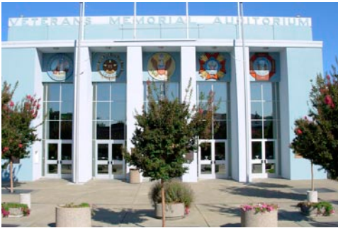
Veterans' Memorial Building, Santa Rosa, California
